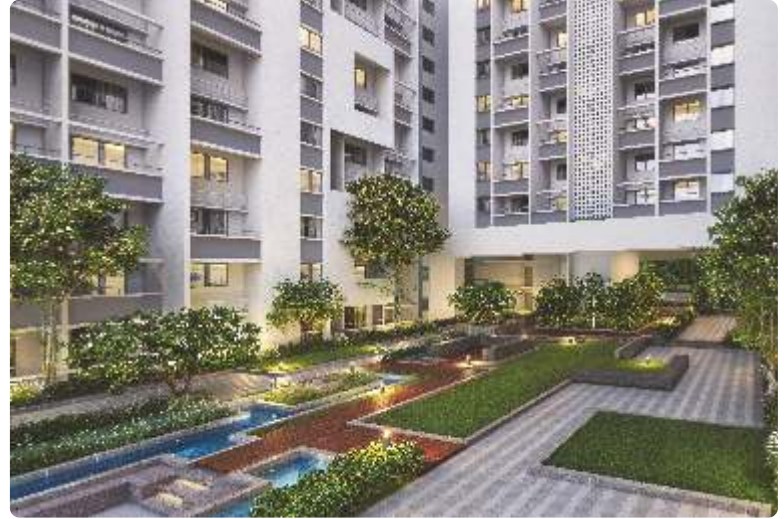
Rohan Prathama, Hinjawadi Phase-1
