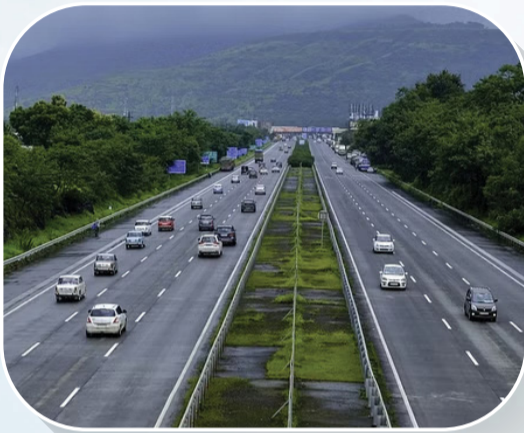
Pune-Bengaluru Highway (NH 48)
