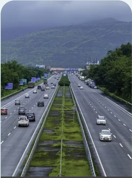
Pune-Bengaluru Highway (NH 48)
